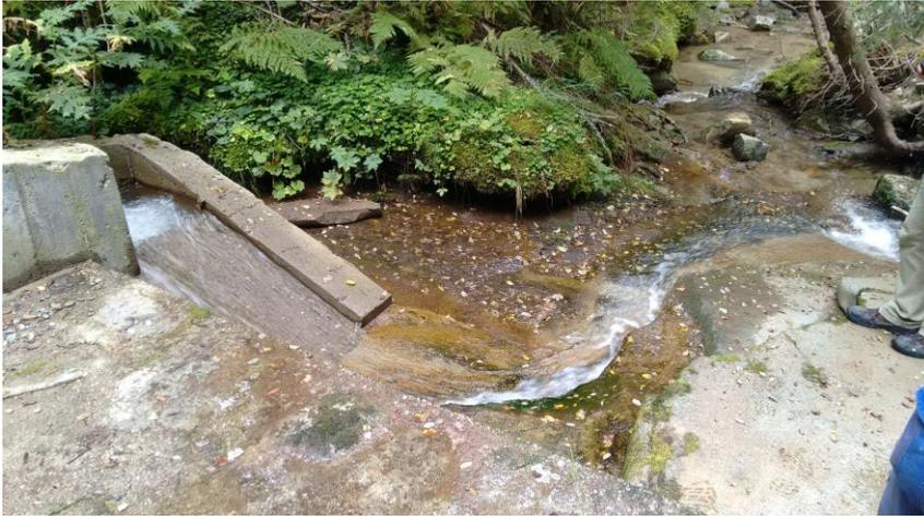
**Figure 8. Existing pool pass – downstream hydraulic connection with the natural river bed**
