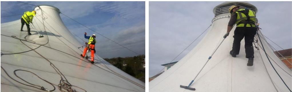
**Figure 2. Cleaning of the membrane structure**
