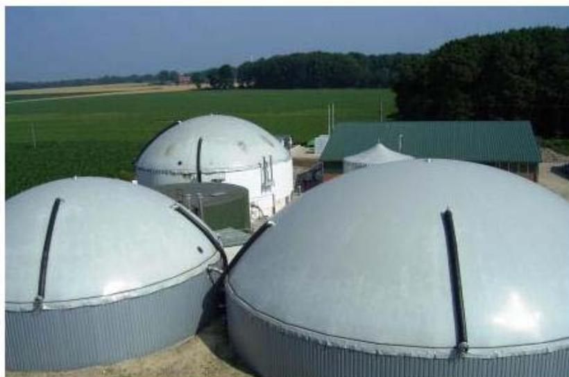
fig. 9 Roof domes from flexible membrane
