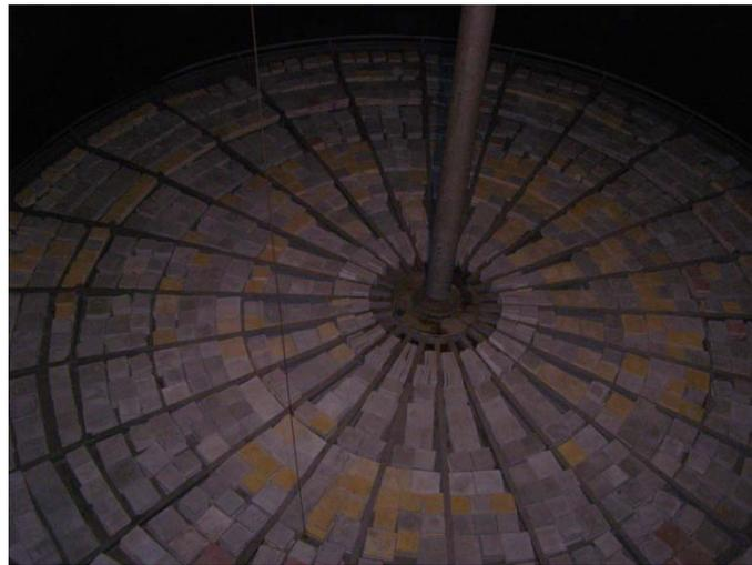
fig. 3 Floating roof with central standing
