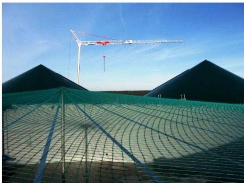
fig. 10 Grate supporting the dome
